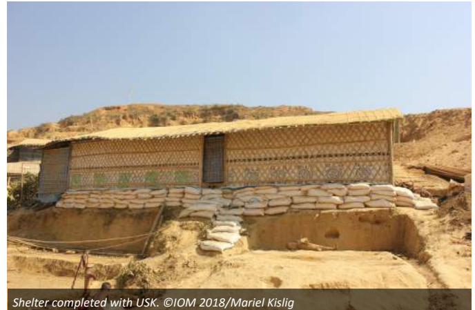
Shelter completed with USK. ©IOM 2018/Mariel Kislig
