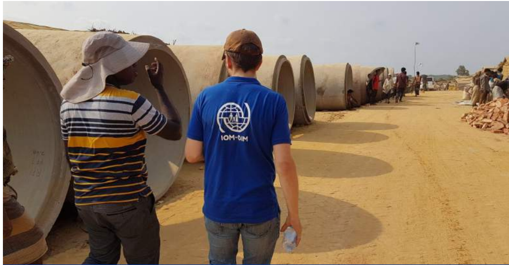
Over 100 culverts have been received and will be installed on Army road in the coming months. © IOM 2018/Fanny Renard
