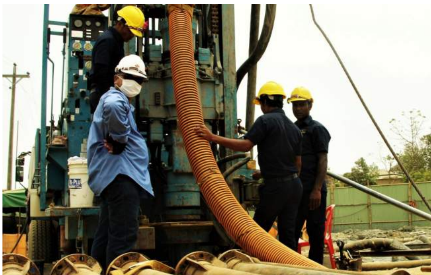
Borehole drilling as part of the joint IOM, JICA, DPHE project in Camp 12.
