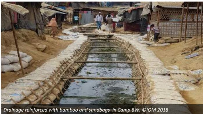
Drainage reinforced with bamboo and sandbags in Camp 8W. ©IOM 2018
