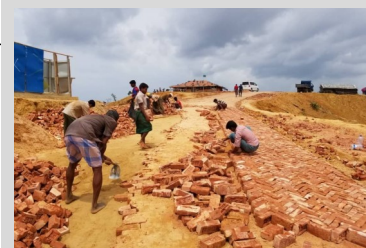
Pavement of Football Field Road Extension.
