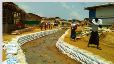
Reinforcement of drainage channels are ongoing.
