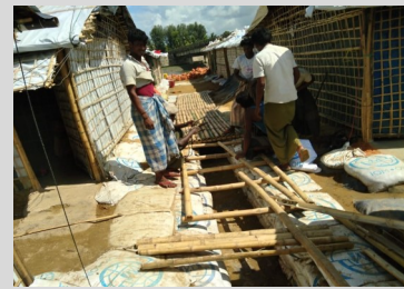
Hatkhula main drainage canal is being covered with bamboos (picture).
