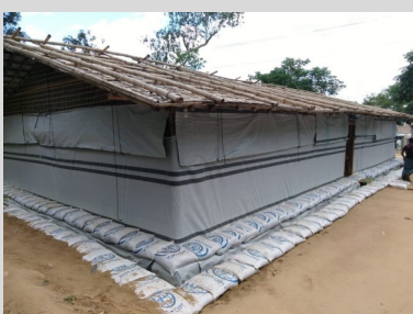
Renovation of Police Camp #4 in Camp 9
