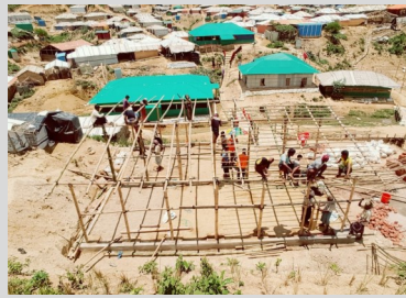
Construction of Camp in Charge (CiC) office in Camp 8W.
