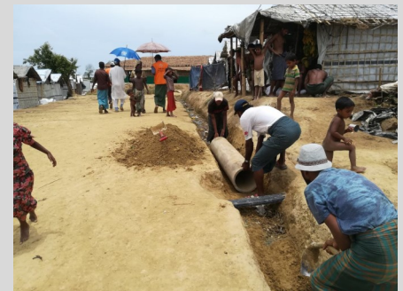
Drainage is also being constructed in the relocation site (picture).
