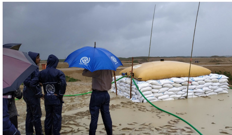
Emergency water supply system was installed in Camp 20 extension.
