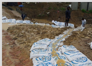
Water diversion channel at UB3 inlet side to protect culvert head wall from seepage and soil erosion.
