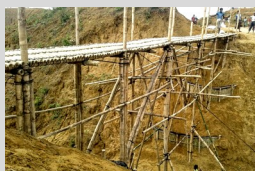
Construction of a bridge connecting two blocks in Camp 20 Extension.
