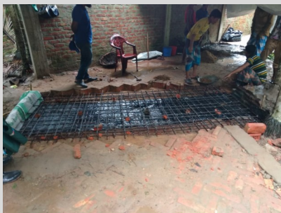
Drainage culvert installation in Noya Para in (Shamlapur).
