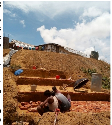
Ongoing Dislodging Tank construction in Camp 20 Extension. @IOM 2018/Rigan Ali Khan
