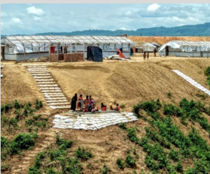
Step and side protection for IOM Deep Tube Well (DTW) in Camp 20 Extension.
