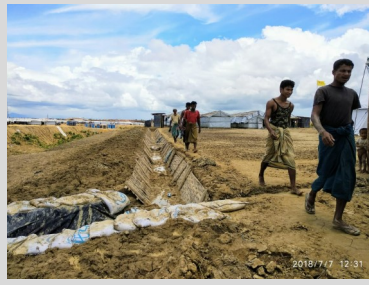
Completed pathway (left) and catch drain improvement (right) in Camp 20 Extension.
