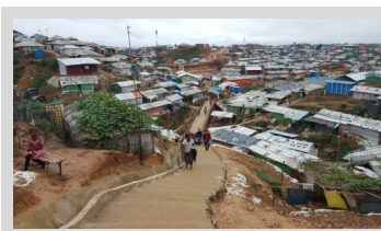
Routes for porters were reinforced with concrete steps and side drain as well as 20m span bamboo bridge.
