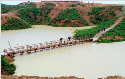
Water level almost reached an IOM bridge after last week rains.
