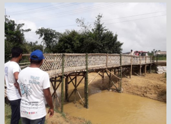
Completed 24-meter bridge in Camp 9.
