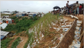
Vetiver grass planted by IOM to retain slopes has grown twice the size in Camp 18.
