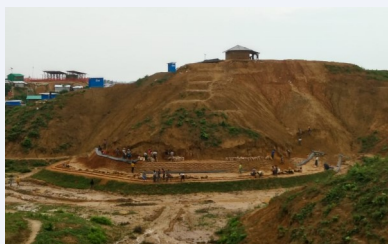
Camp 20 Special Project with earth terraces for shelter and grass turfing
