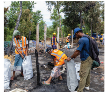
Debris cleaning from the fire affected area. ©IOM2024
