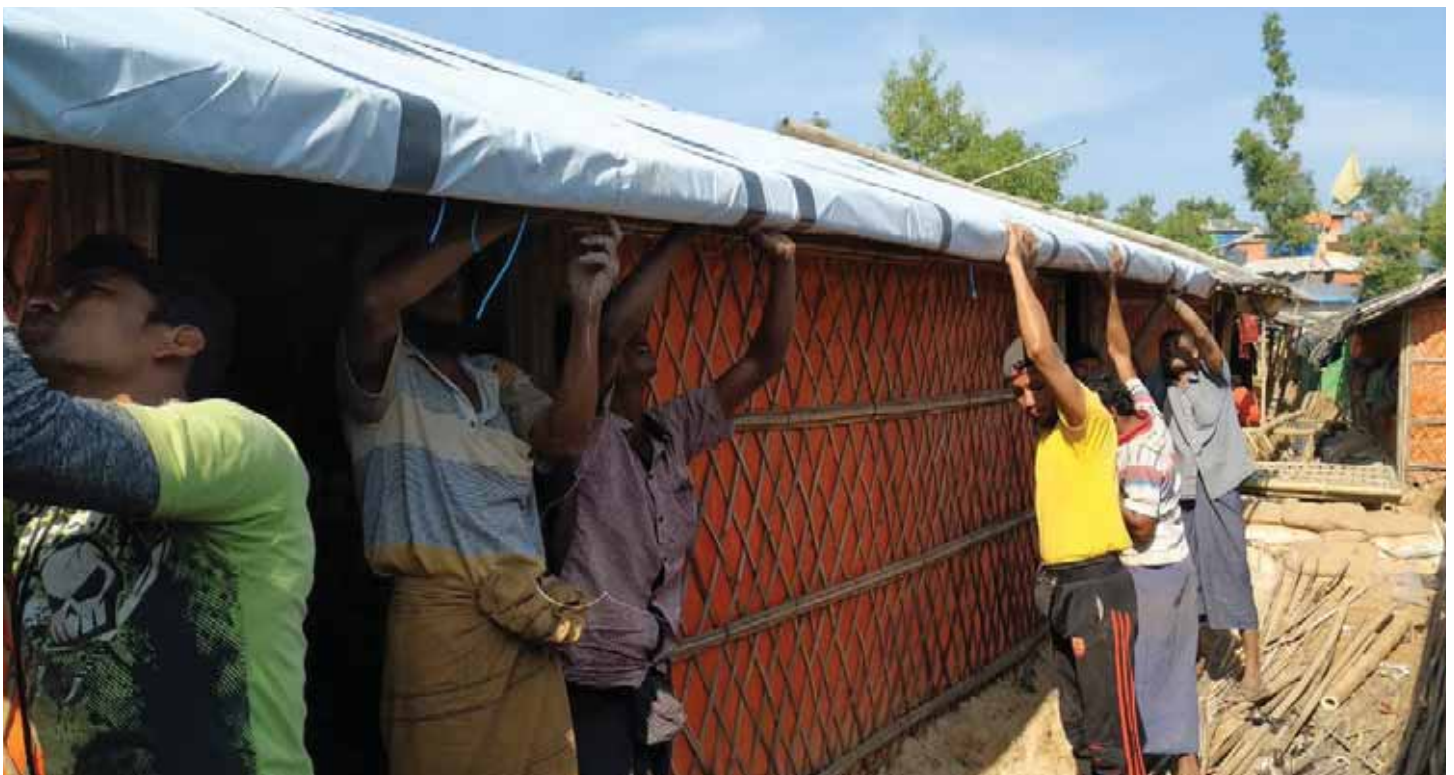
SHELTER IS BEING UPGRADED USING BAMBOO TREATED AT IOM FACILITY © IOM 2018
