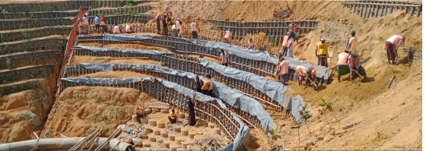
SLOPE STABILIZATION FOR COVID-19 HOSPITAL IN CAMP 20 EXTENSION © IOM 2019
