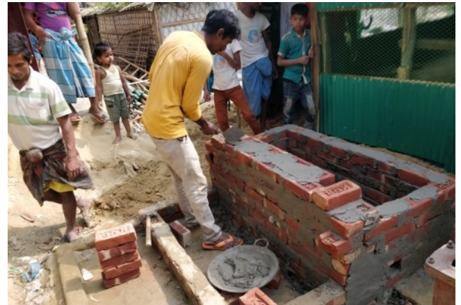
CONSTRUCTION OF PLATFORM FOR TAP STANDS OF WATER PIPELINE NETWORK. ©IOM 2019
