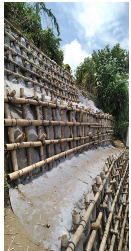
STABILIZATION SLOPE WALL INSTALLED BY SMEP TEAMS IN CAMP 22 © IOM 2020
