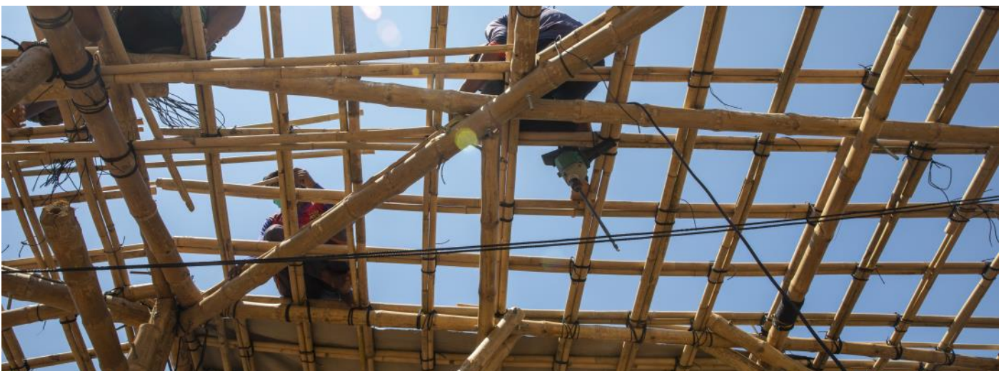
CFW BENEFICIARIES CONSTRUCT ROOFING FOR LEDA ITC © IOM 2020
